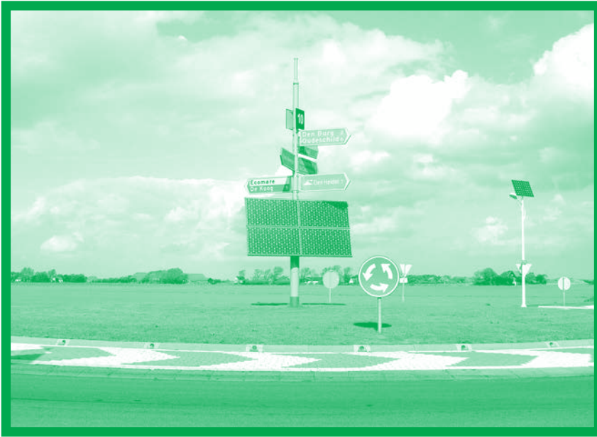
A roundabout on Texel fitted with solar panels. Source: voordevereldvanmorgen.nl
