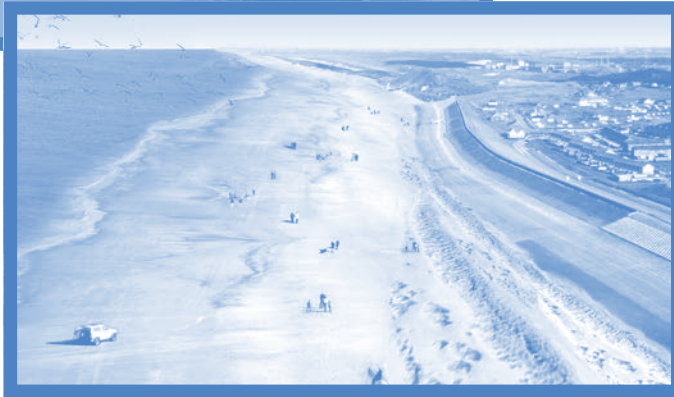
As a result of sand supplementation, the Hondsbossche Zeewering gains a beach and Petten is able to grow into a coastal resort. Photo: new landscapes, Miranda Reitsma / PARK
